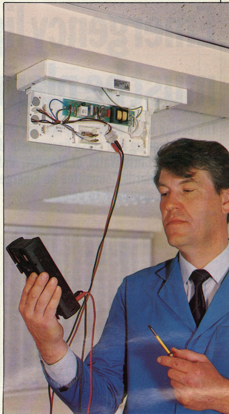
A maintenance engineer testing the voltage of an emergency light fitting.
